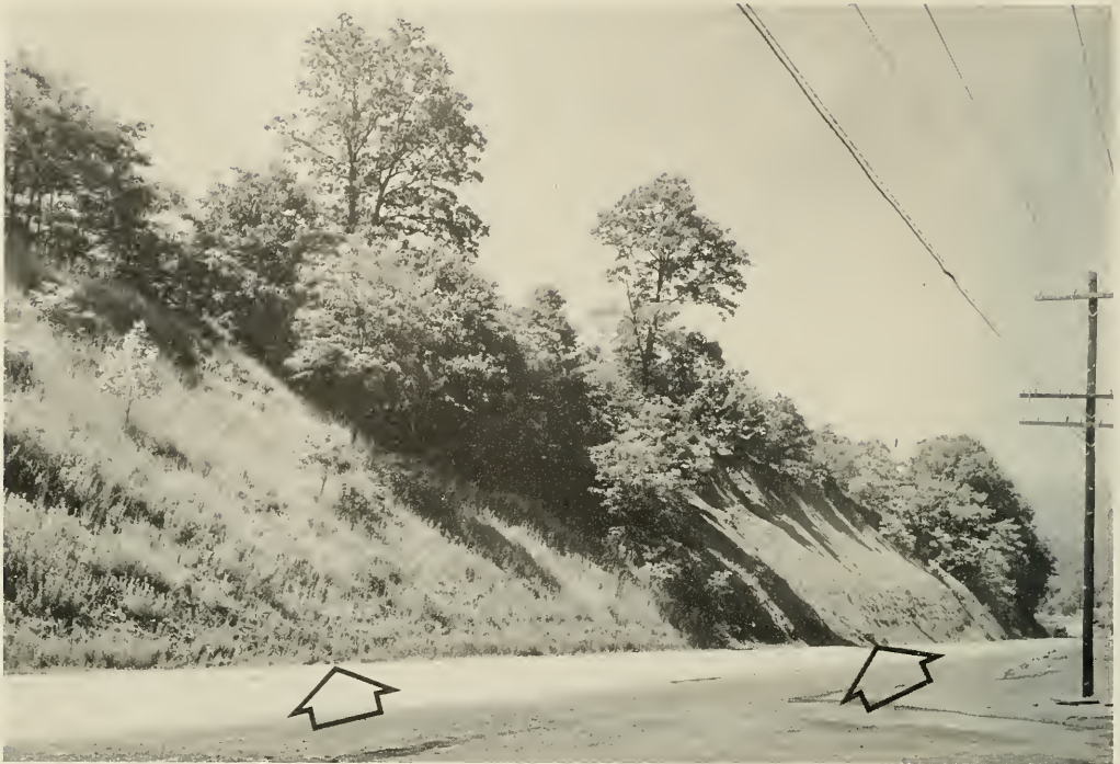
BARE ROADBANK AT RIGHT WILL ERODE EASILY, BUT VEGETATION-COVERED BANK AT LEFT WILL HOLD.
